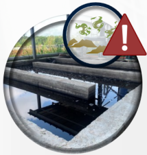
Boiler wet scrubber system
